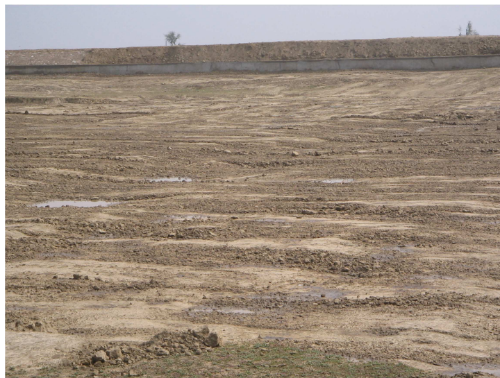
Pond site after the excavation work
