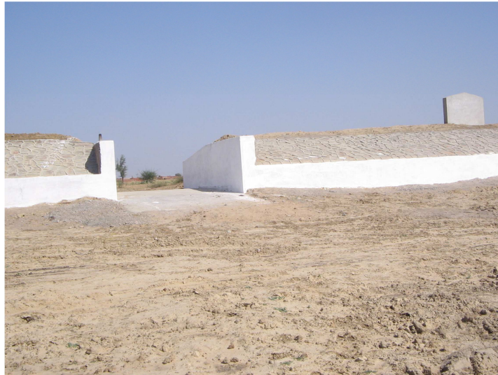
Overflow and Face-wall structure of the pond
