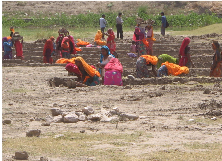
Excavation work carried out by villagers
